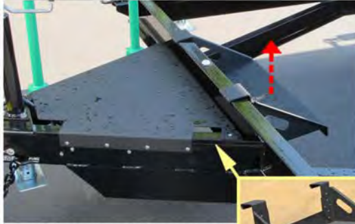
Installing additional staircase
